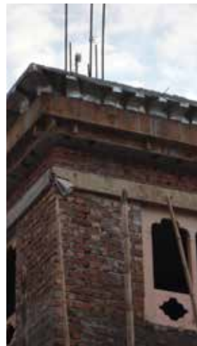
Focus on cheap and fake imitations of traditional construction: painting on concrete construction in Thimphu and wood replacement by using concrete elements in the new Wangdue town
