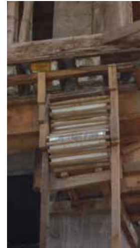
Focus on cheap and fake imitations of traditional construction: painting on concrete construction in Thimphu and wood replacement by using concrete elements in the new Wangdue town
