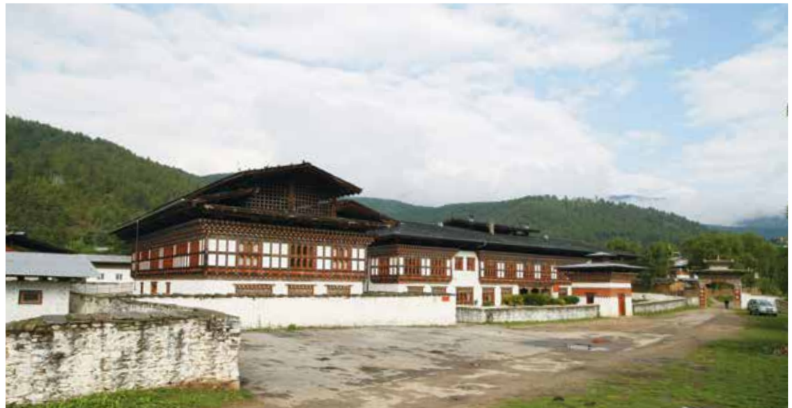
Wangdichoeling Hospital with main entrance
