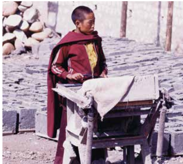
Cement Hollow Block production
