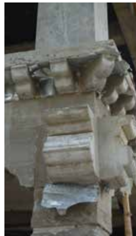
Focus on cheap and fake imitations of traditional construction: painting on concrete construction in Thimphu and wood replacement by using concrete elements in the new Wangdue town
