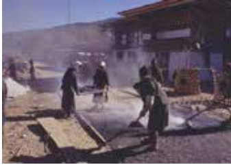
Wangdichoeling Hospital, first phase of construction
