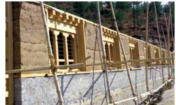
Rammed earth and wooden window frames
