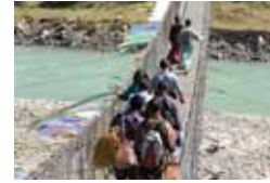
Punakha suspension bridge, photo: Markus Wild
