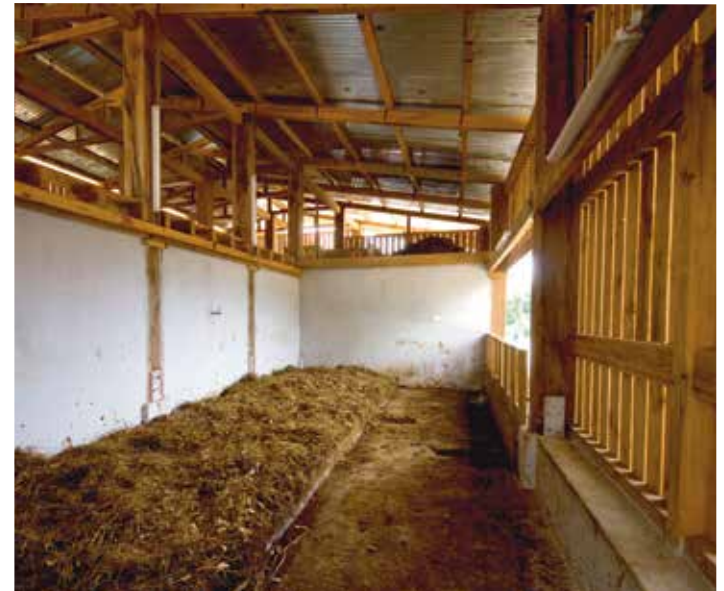
Cattle shed, interior view
