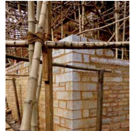
Stone masonry wall construction
