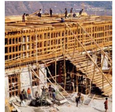
Ekra wall and roof construction
