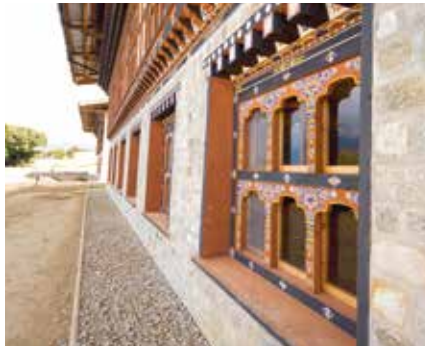
Facade of school building
