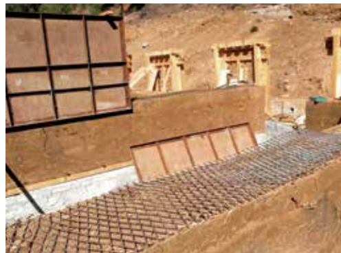
Rammed earth construction with expanded metal sheet
