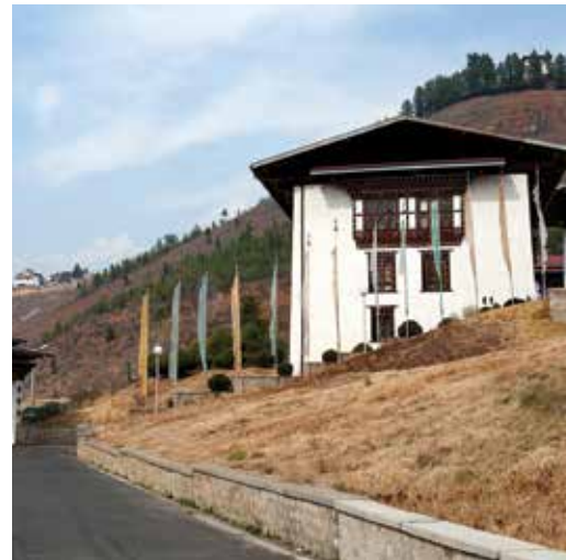
Road and stonewall following the natural topography
