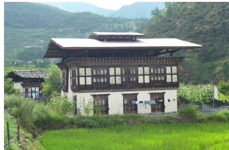
Houses in Paro with Jamthok roof (Picture: Dorji Yangki)
