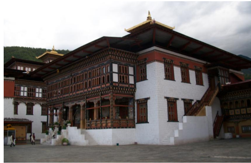
Chenkhep roof over Rabsel at Kunrey of Trashichodzong in Thimphu (Pictures: Dorji Yangki)
