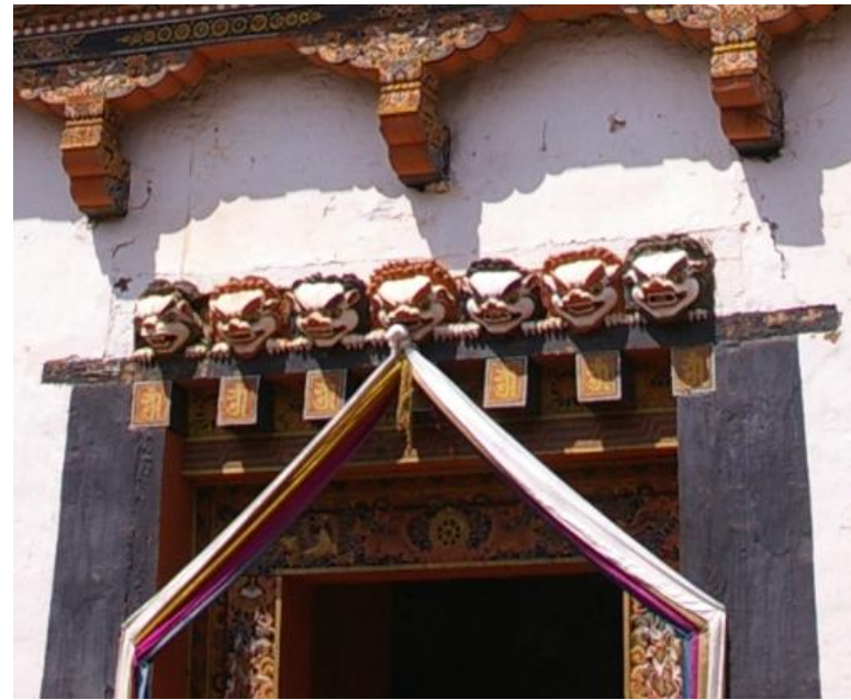
Mythical Snow Lion heads carved in timber placed above the main Mago door to a Lhakhang
