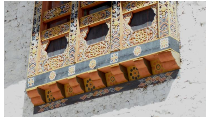
Tshechu Kha-nyim with embedded Dhung and without Pem Choetse below Rabsel window at Semtokha Dzong
