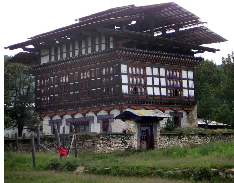
A typical Bhutanese layered “flying roof” in Bumthang (Picture: Dorji Yangki)
