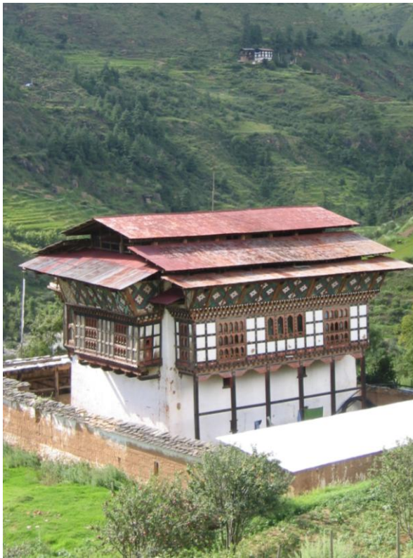
Chenkhep roof over Rabsel of a House in Thimphu
